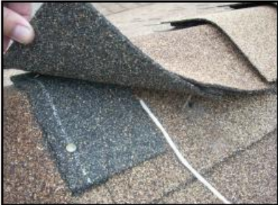
FIGURE 2 DRILL HOLE UNDER RIDGE
